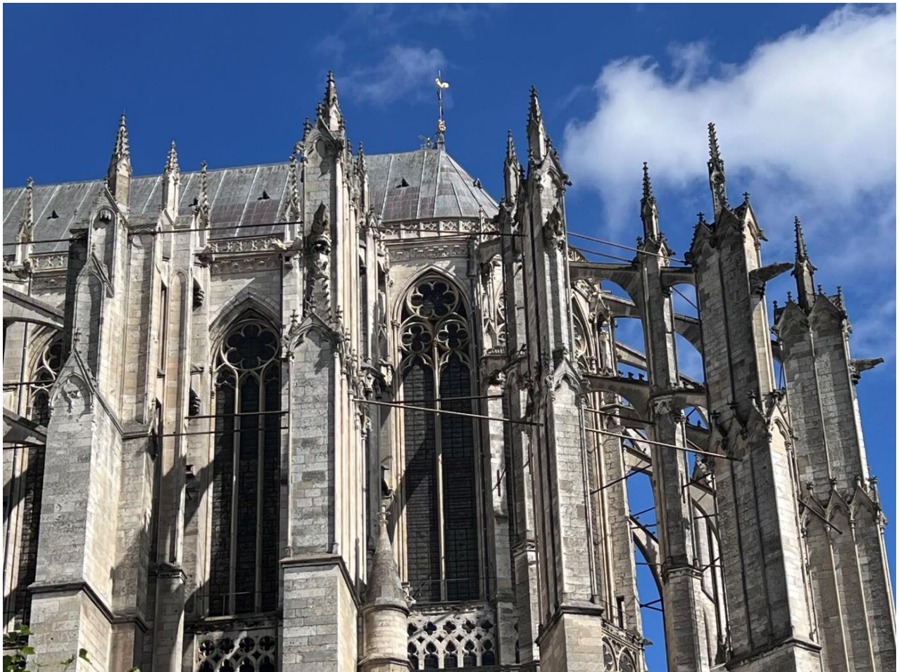
Figure 3. View of the apse from the south side showing buttresses and iron tie-rods connecting them (photograph by the author).
