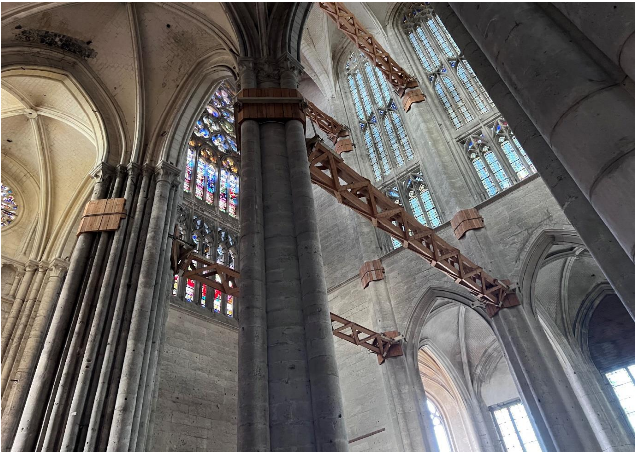
Figure 2. Interior view of Beauvais Cathedral showing transept piers, wooden tie beams, and stained-glass windows (photograph by the author).
